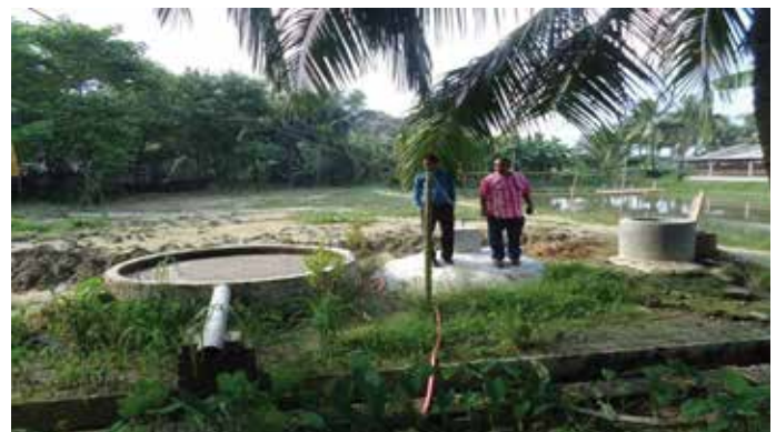
Bio-gas Plant of M/S. Z. H. Agro Park at Comilla District under Process for Financing by SBL, Comilla Branch.
